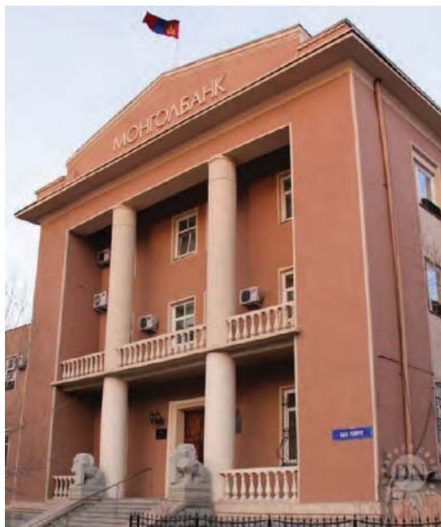
Front view of BOM building
